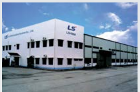
Hanoi factory (Vietnam) MV/LV switchgear, Mold TR
