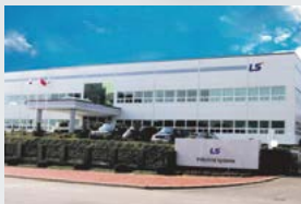
Dalian factory (China) MV/LV switchgear, MV contactor
